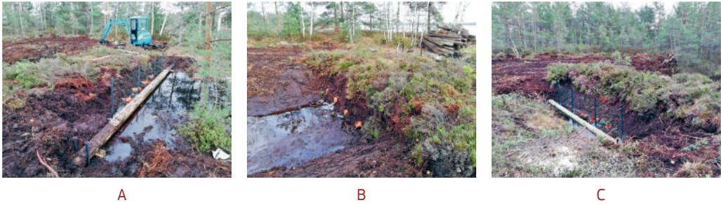
Figure 174. Construction of peat dams in Lauga Mire. Photos: G. Šusts.
